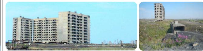
Figure 3. Left: Building constructed using piling foundation on permafrost. The piles can also be seen on the right from the building. Various heights of the piles shows differential frost heave processes over the construction site. Right: underground utility collector. The heat excess from a network of such collectors is one of the main reasons of permafrost degradation in urban areas, such as shown on Figure 1 for Norilsk (Photo by D. Streletskiy, July 2013.)
